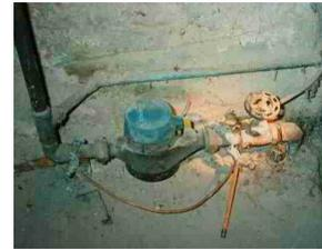
Photo of a damaged grounding electrode to a water pipe at an industrial plant.
