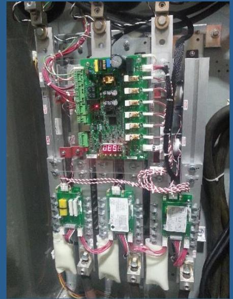
*Adjustable speed drives can be threatening to LED lighting if not properly powered and grounded.*
